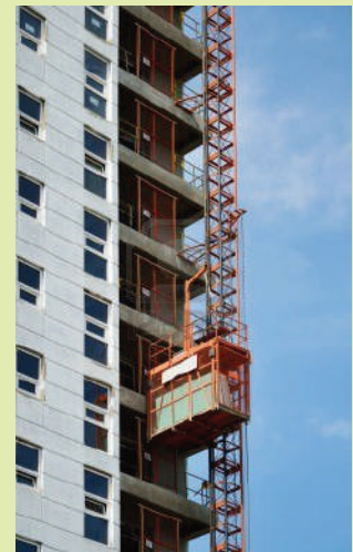
Lift to take materials
